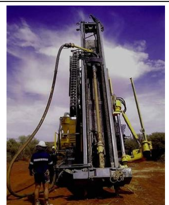
Drilling machine for exploration 勘探用鑽孔機
